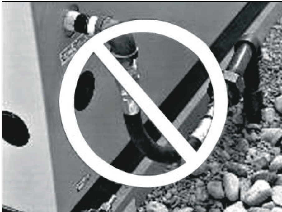
Figure 5-4. Incorrect Routing of Flexible Hose
