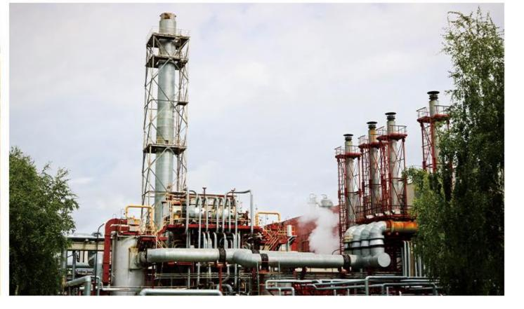
Fuelled by natural gas, the 4MW plant generates electricity and heat, making the best possible use of the energy from CHP. With well proven CHP technology, it contributes to the financial and carbon savings through its high efficient use of energy, which provides a good return on investment.
